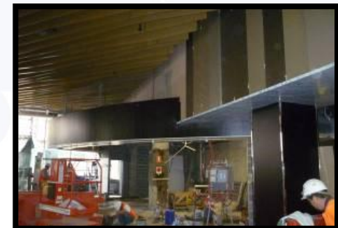
Steelwork at Level 5, Centre Point Tower
