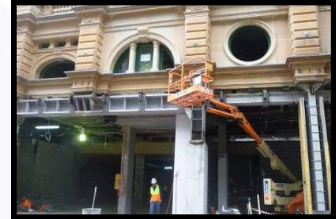
Beams on Pitt St entrance
